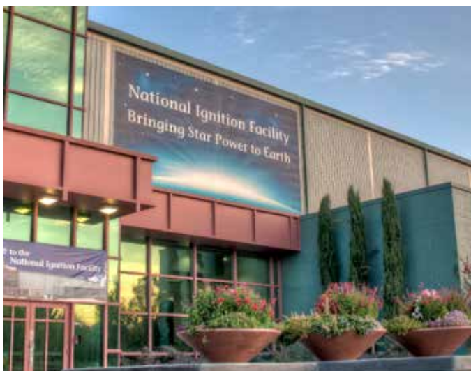
▲ Lawrence Livermore’s National Ignition Facility is 10 stories tall and as wide as three football fields. Its main entrance is pictured here. Photo: LLNL/Jason Laureia
